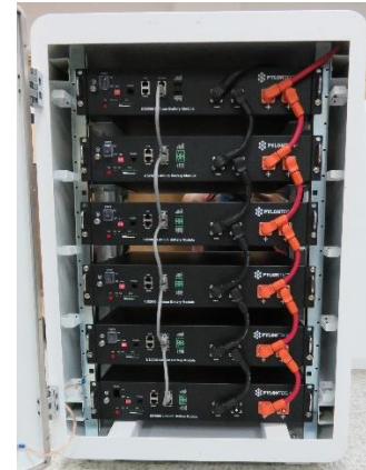
Fig.7 Linking Of Batteries
