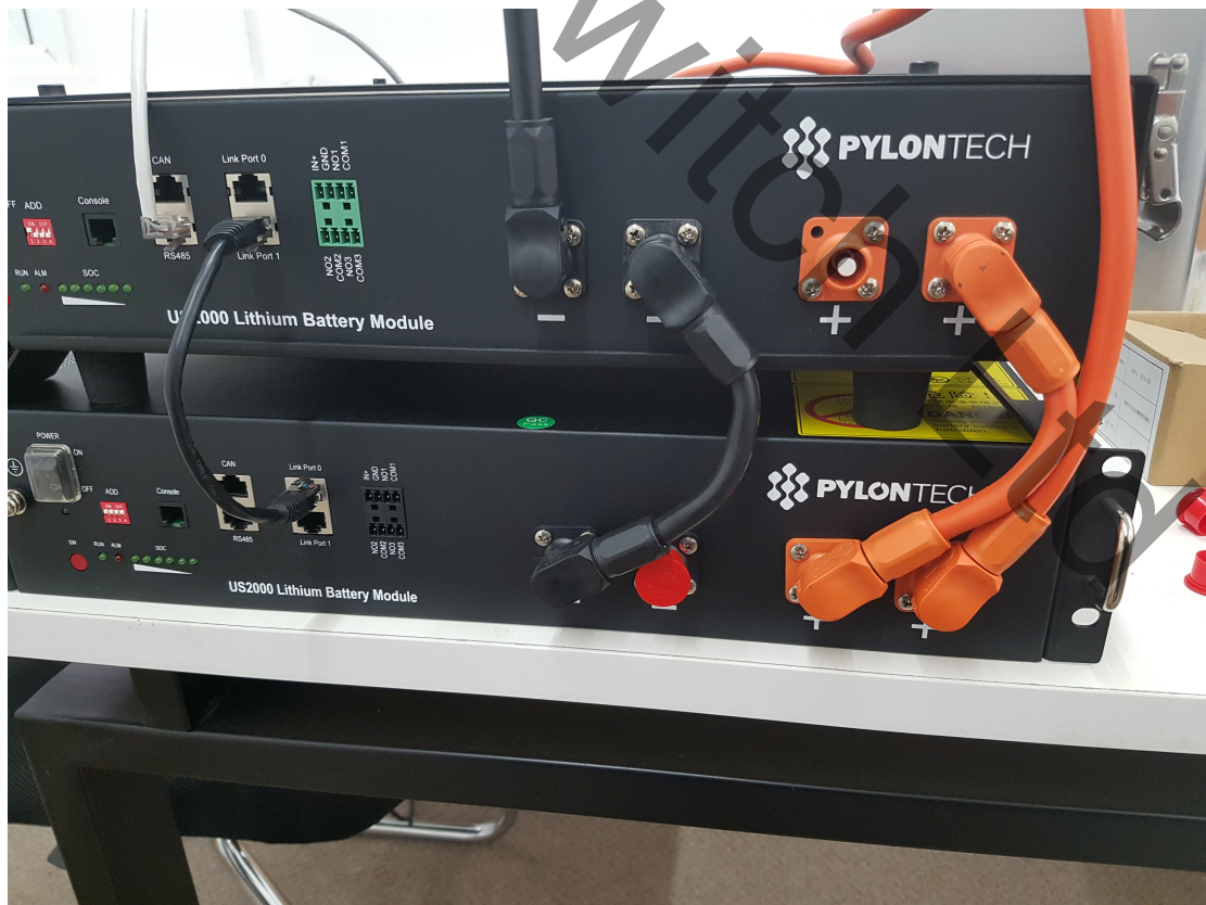
Fig 8. Long Power Cable Connection to ME3000SP
